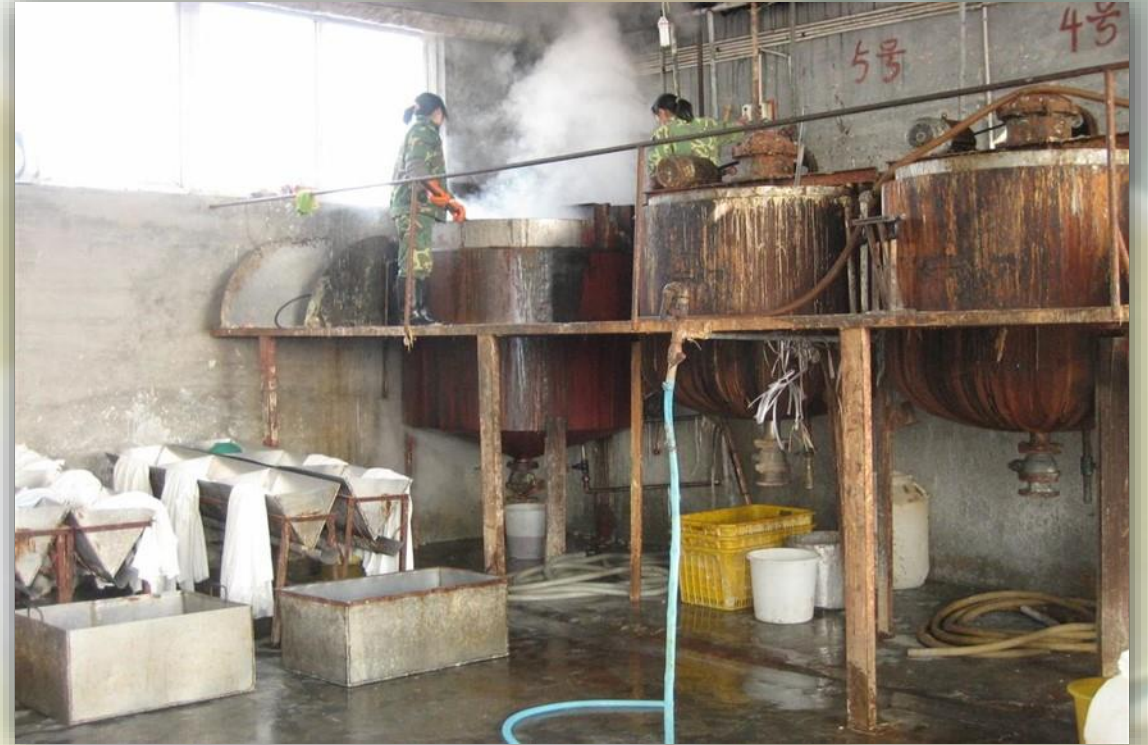
Non Compliant Reactors
